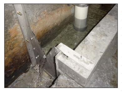
Geosense® V-Notch Weirs and Tanks are used to measure seepage water flows in open streams, channels or tanks and are used mainly as part of Dam Safety Monitoring programs.
